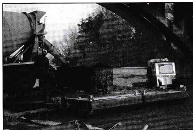
Loading concrete onto a barge under the QEW bridge
