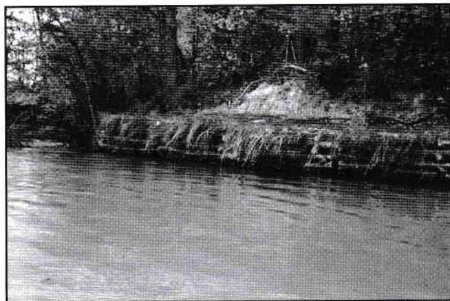
Timber cribs forming erosion protection
