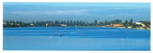
The late 1970s saw the design and construction of a course buoying system that, along with pontoons for a held start, and a stretch of water eight lanes wide, 2400m long and at least 3.5m deep, enabled the course to gain FISA accreditation. This qualified the course and on shore facilities to be considered for national and international events such as the World Masters Rowing Championships held on the course in 1997.
